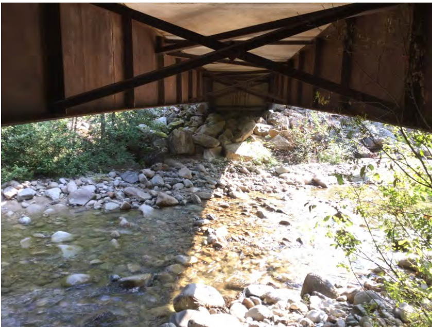
Right Bank Abutment when facing downstream
