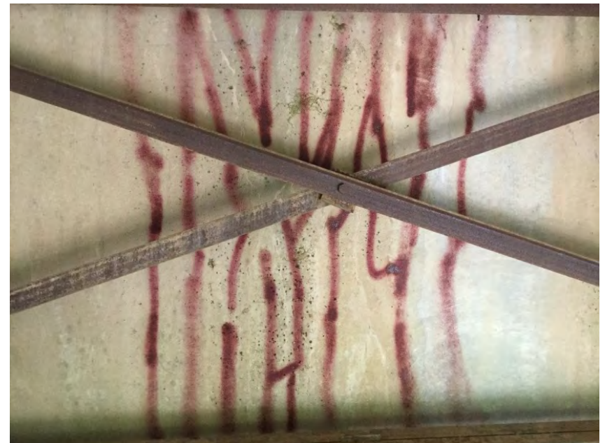
Hairline cracks noted on right bank ballast wall
