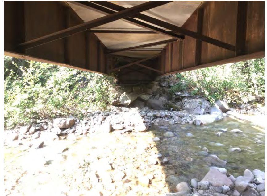
Left Bank Abutment when facing downstream
